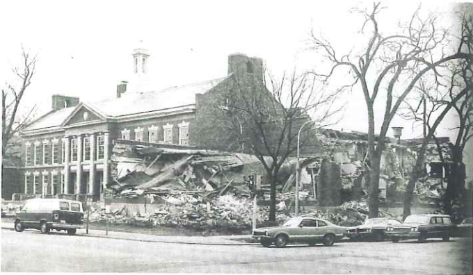
Demolition begins on Lowell School early in 1973
