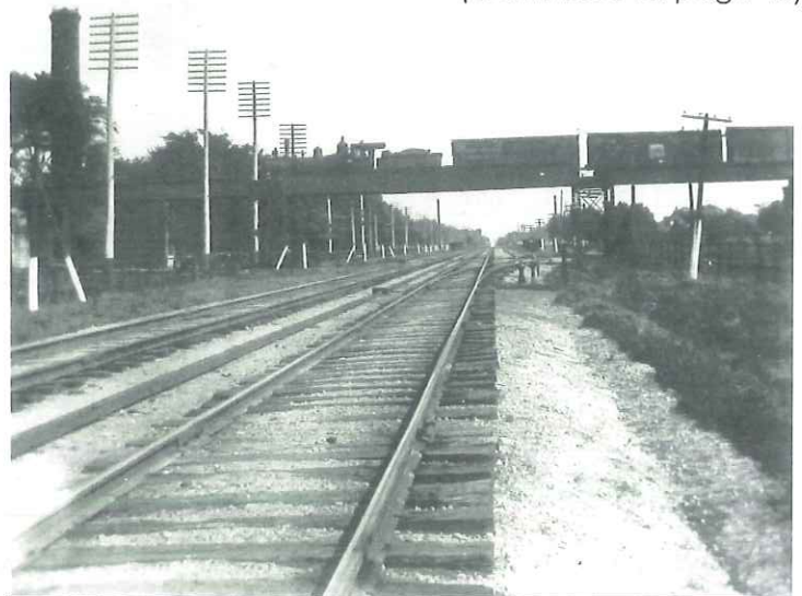
Soo Line viaduct shown above what are today the Metra tracks (formerly C&NW Railroad) east from Keystone in about 1905.
